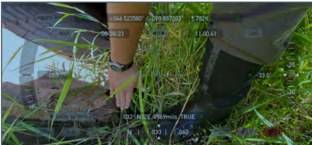
Photo of Beartrap Creek culvert at Hegstrom Rd; MNRD Staff, 2023.
